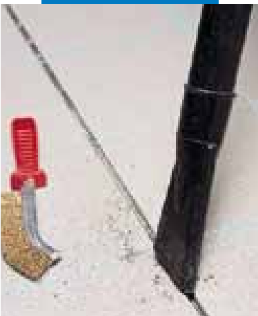
Cleaning out the joint with a vacume cleaner
