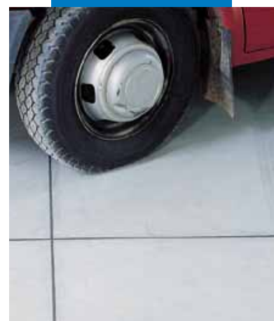
Movement joints of an industrial concrete floor sealed with Mapeflex PU21
